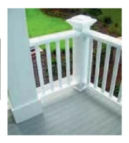
An AZEK Rail kit contains everything needed to assemble a section of railing (top rail, bottom rail, balusters, etc.) and hardware to attach the railing sections to the posts. Rail kits
